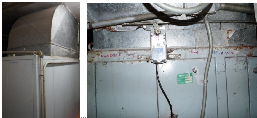
Servomotor clapetas aire
